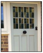
6. Visable double reflection can occur under certain lighting aspect conditions, especially when viewed from an angle. This is an optical phenomenon arising from multiple surface reflections in sealed units.
