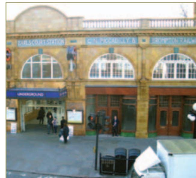
Earls Court Station, London.
